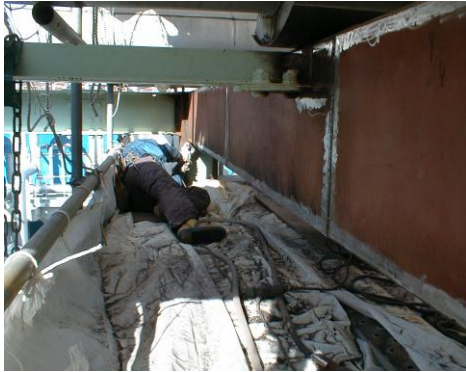
Photograph -7 The earthquake-proof reinforcement work
