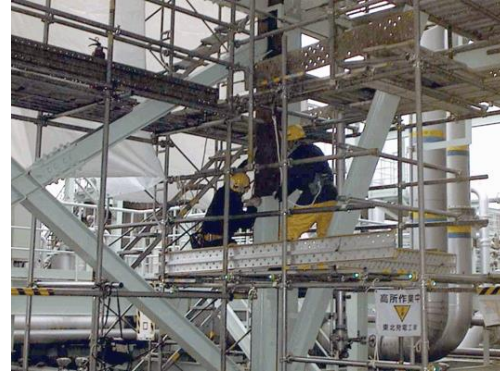
Photograph -8 The earthquake-proof reinforcement work
